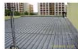
2) Class Room 4.8 - Metal Roof area - approximately 103m 2
