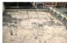
1) Staff room - Concrete Roof area - approximately 360m 2
